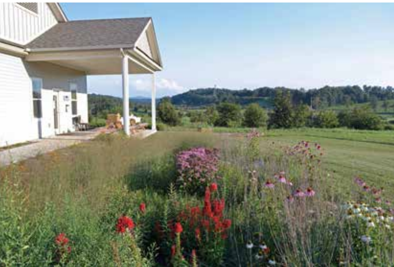
The Meadowview rain garden with the Price Laboratory and Meadowview chestnut orchard in the background.
