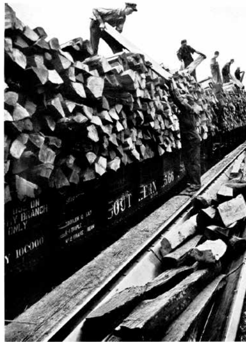
Two hundred and seventy-five cords of chestnut from timberlands or woodyard reserve are carried along this ramp into the extract plant each twenty-four hour working day.
