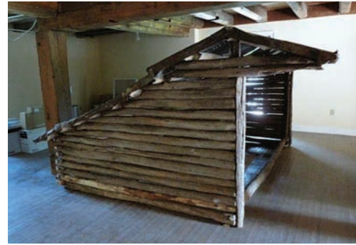
The shelter used by Earl Shaffer, the first thru-hiker on the Appalachian Trail was reconstructed using American chestnut logs. Photo Courtesy of Alex Day
