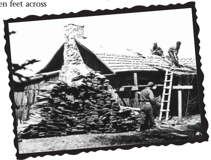
Civilian Conservation Corps workers roof a cabin with chestnut shingles. Courtesy Shenandoah National Park Archives.
